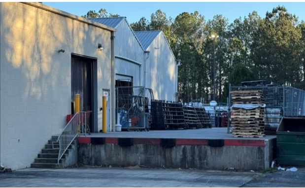
Dock High Landing Docks
